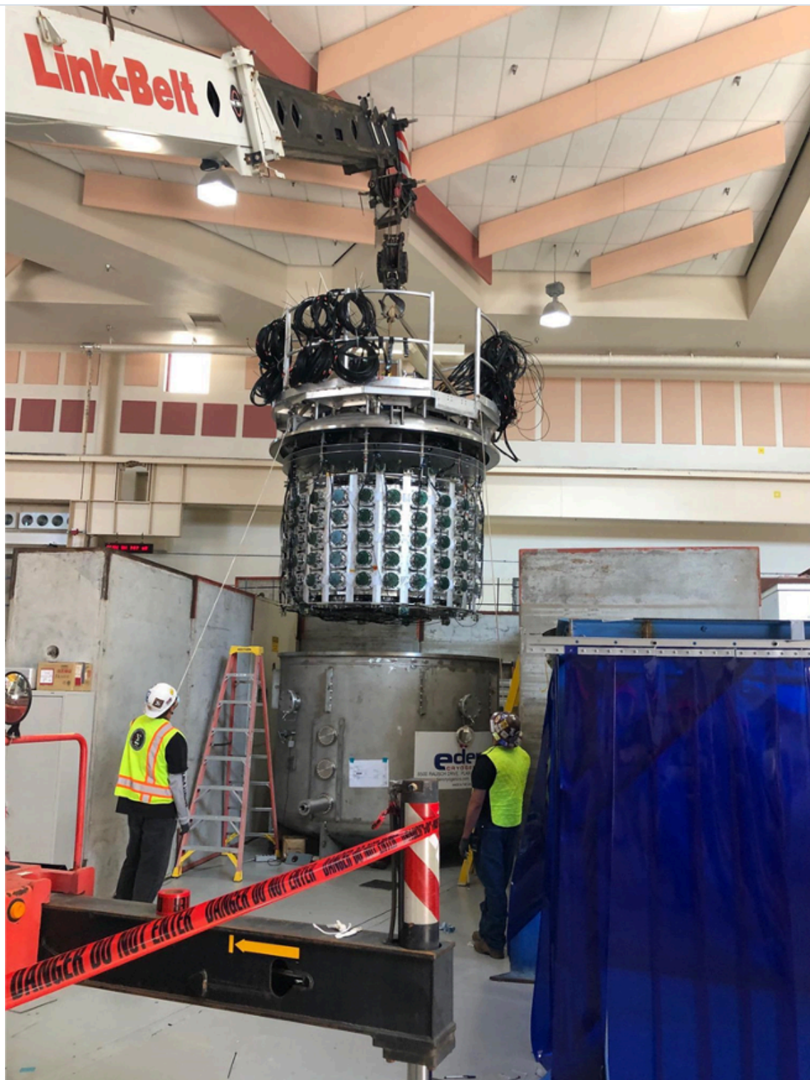
CCM detector installation using a mobile crane inside the Lujan Center experimental building.
